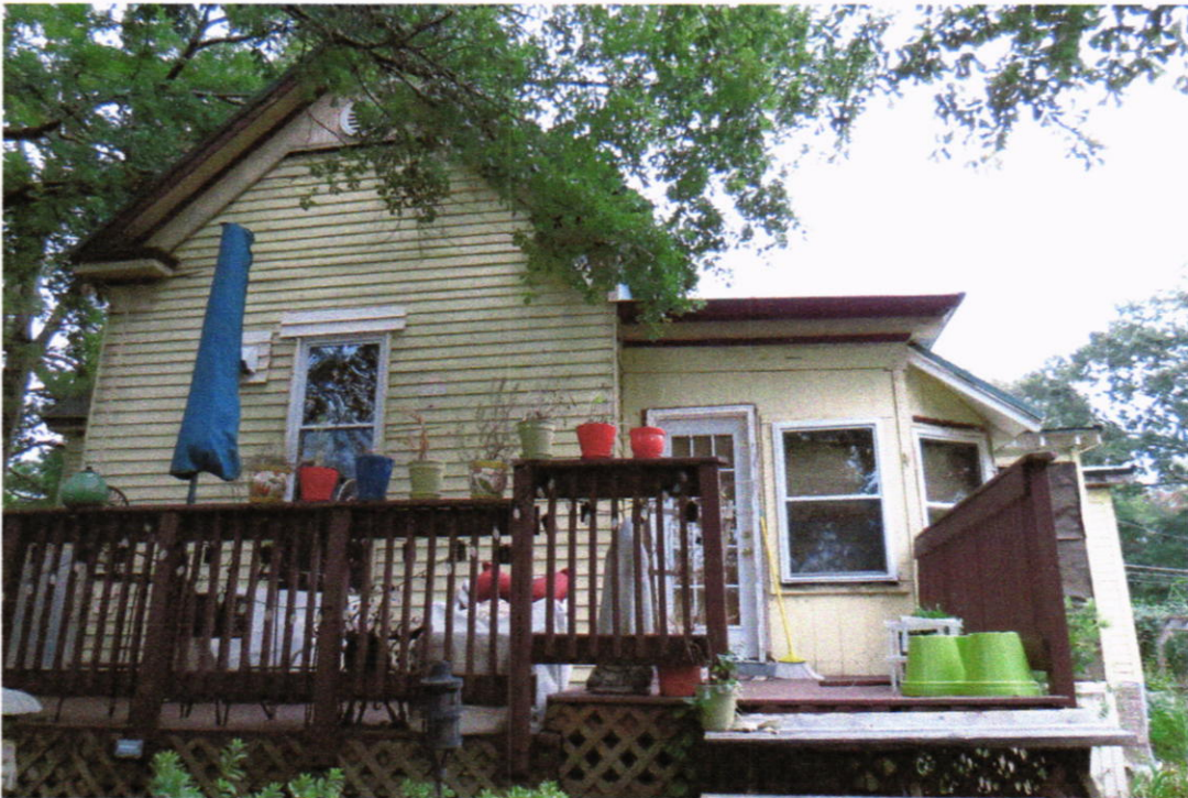
Back of house without siding
