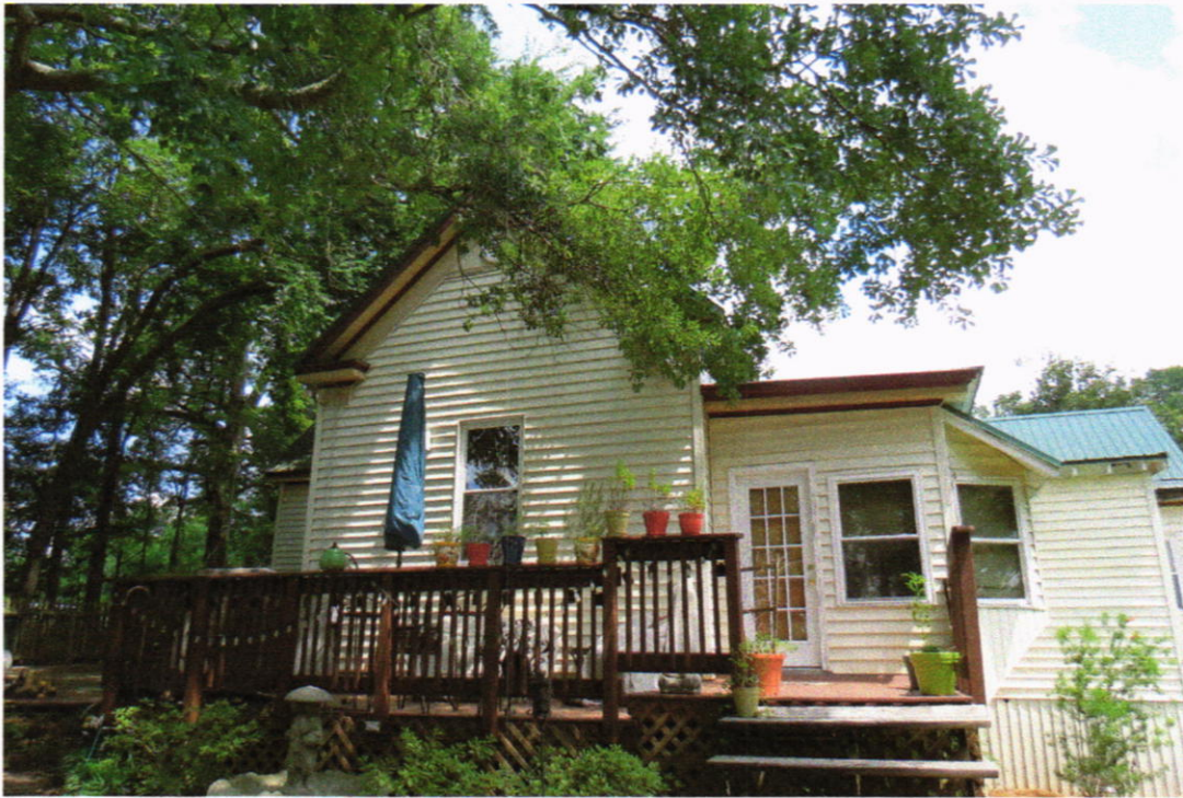
Back of house with siding
