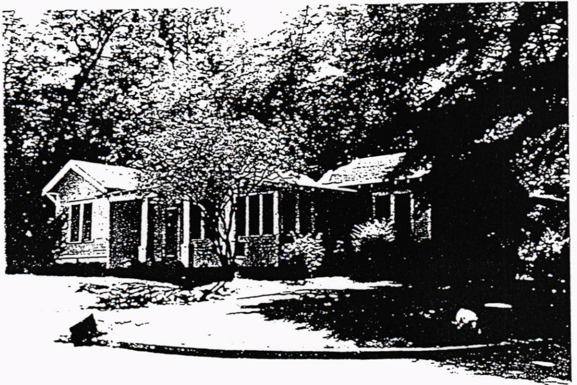
Top: 307 East Main Street Bottom: 109 Landrum Street
