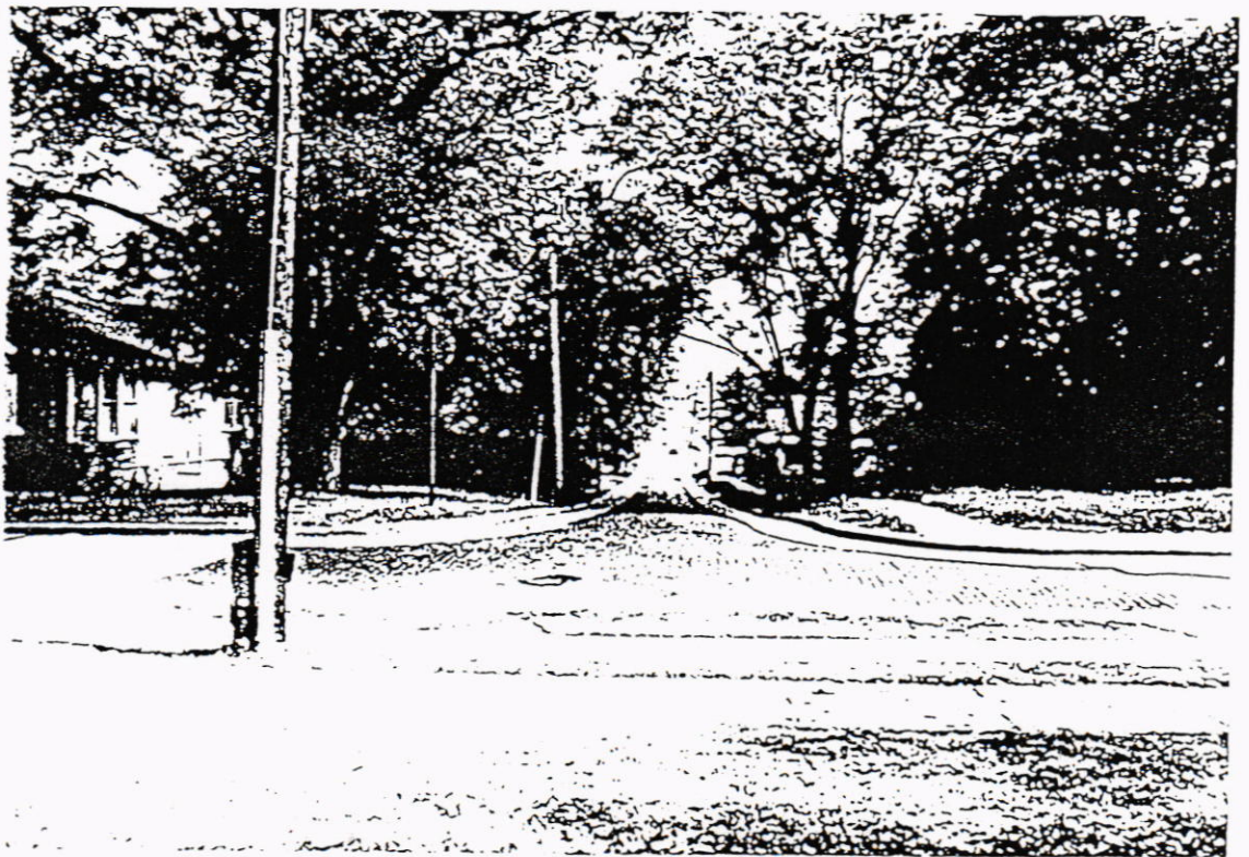
Top 206 East Main Street Bottom: Intersection of East Main St., looking south on New Prospect St.
