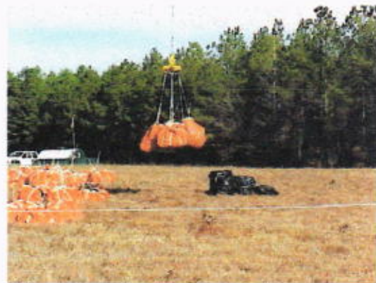
Helicopter moving equipment.
